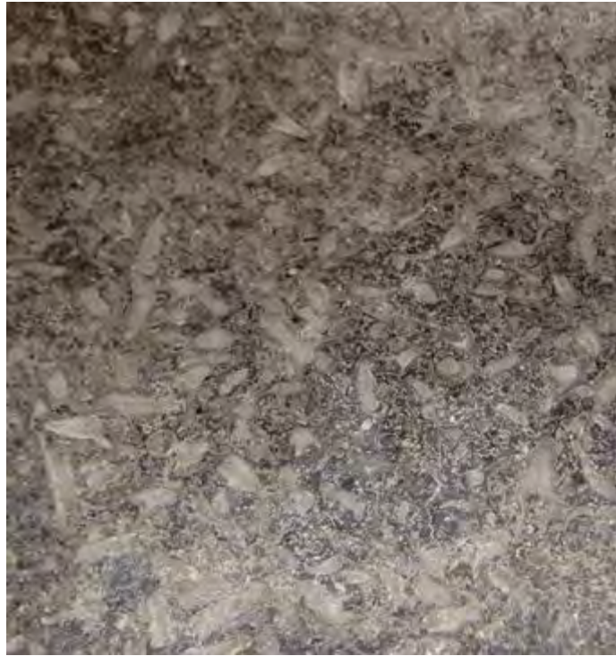
Detail of Marton church chancel step.
