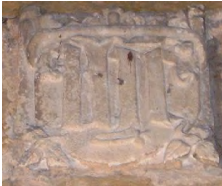
Detail of Marton church tower inside. Note the different style of crown on the top of the shield.
